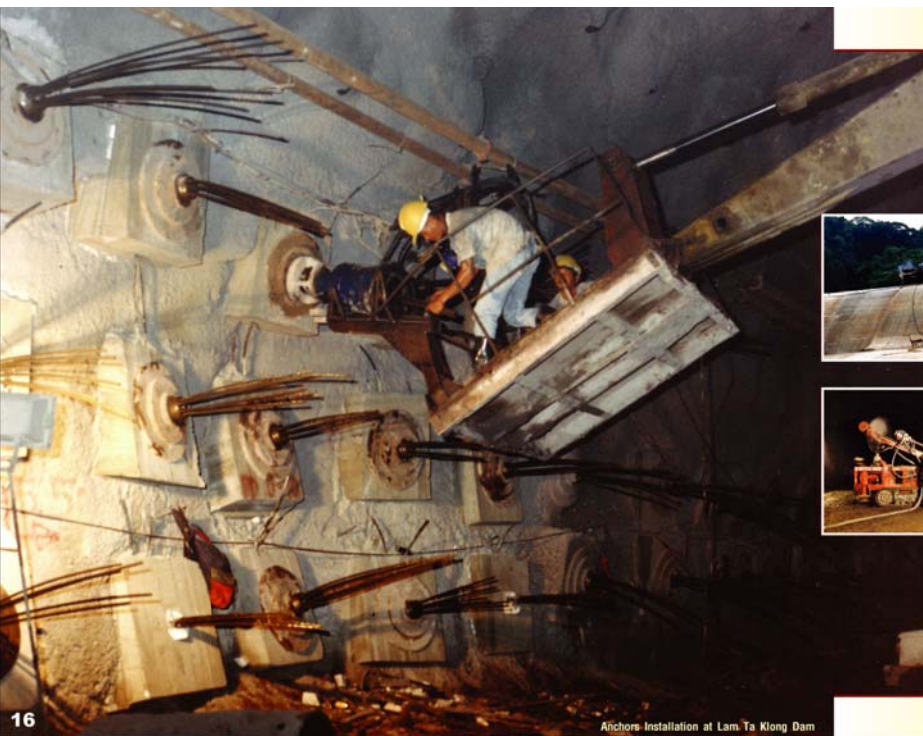
Aichors Installation at Lam Ta Klong Dam
