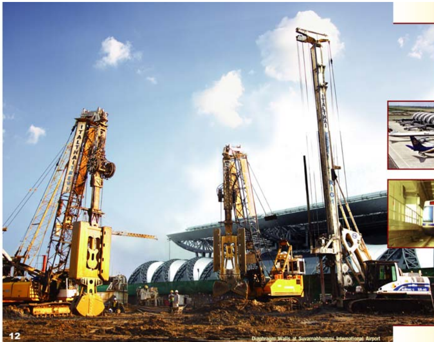
Diaphragm Walls at Suvarnabhumi International Airport
