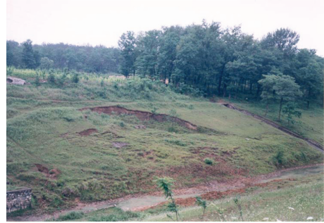
Figure 3. A typical failure of an expansive soil slope at Dagangpo (Zhan 2003).
