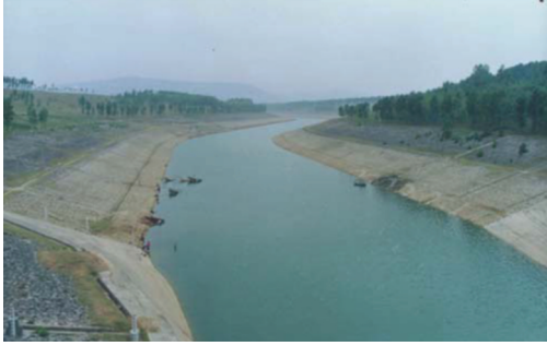
Figure 2. Intake canal of the SNWTP (middle-route).
