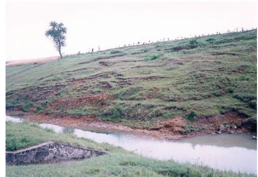
Figure 4. A typical shallow retrogressive slope failure at Dagangpo (Zhan 2003).
